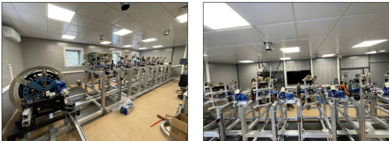
Figure 16. Pictures of the cable/winding machine.
