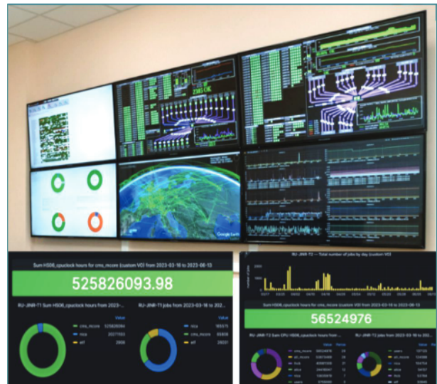
MICC monitoring system
