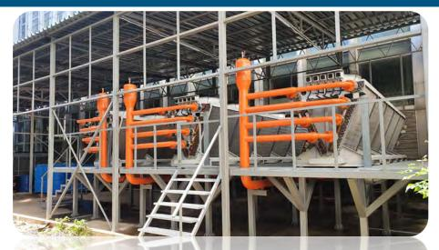
Dry cooling towers of the MICC cooling system
