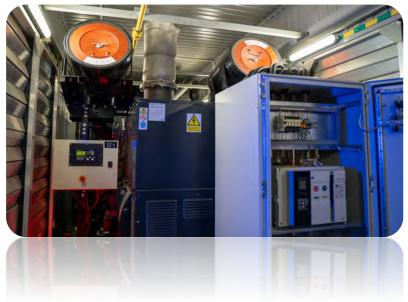
Main tank – 1 ton Additional tank – 2 tons Consumption – 335 l/h at 1 MW Operating time with a full tank ~ 8 h
