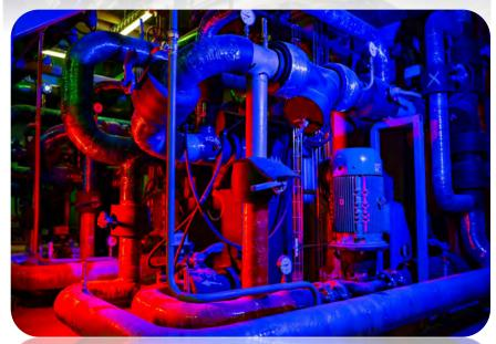
Dry Cooling Tower Pump and Heat Exchanger
